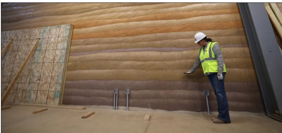
Forum file photo Jenn Carroll, manager of sustainability for the Theodore Roosevelt Presidential Library Foundation, points out the layers of a rammed-earth wall installed inside the library near Medora.
