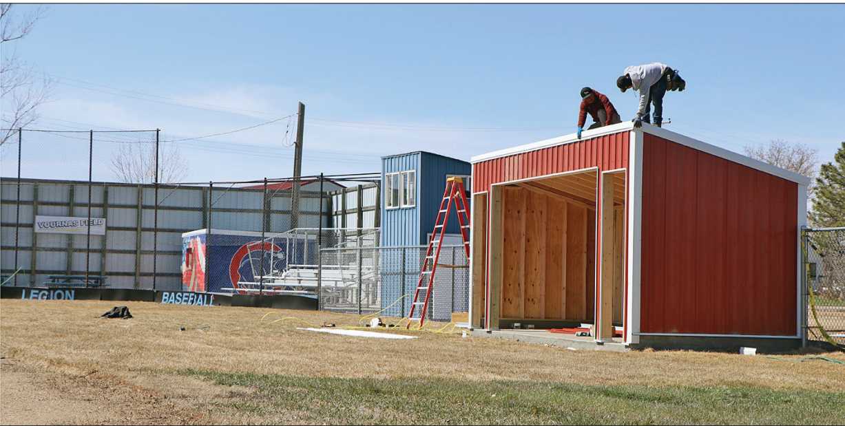
Jody Michael -- The Journal Contractors install the exterior panels for one of the new dugouts under construction at Vournas Field in Crosby on Saturday, part of a larger renovation project for the baseball diamond. The Divide County High School baseball team is currently playing all of its games on the road while the renovations are finished.
